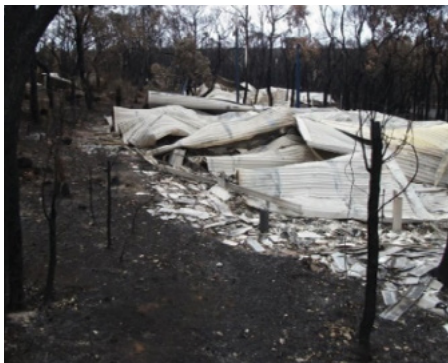
Dwelling destroyed by out-of-control prescribed burn in Margaret River.
