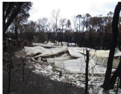
Dwelling destroyed by out-of-control prescribed burn in Margaret River.
